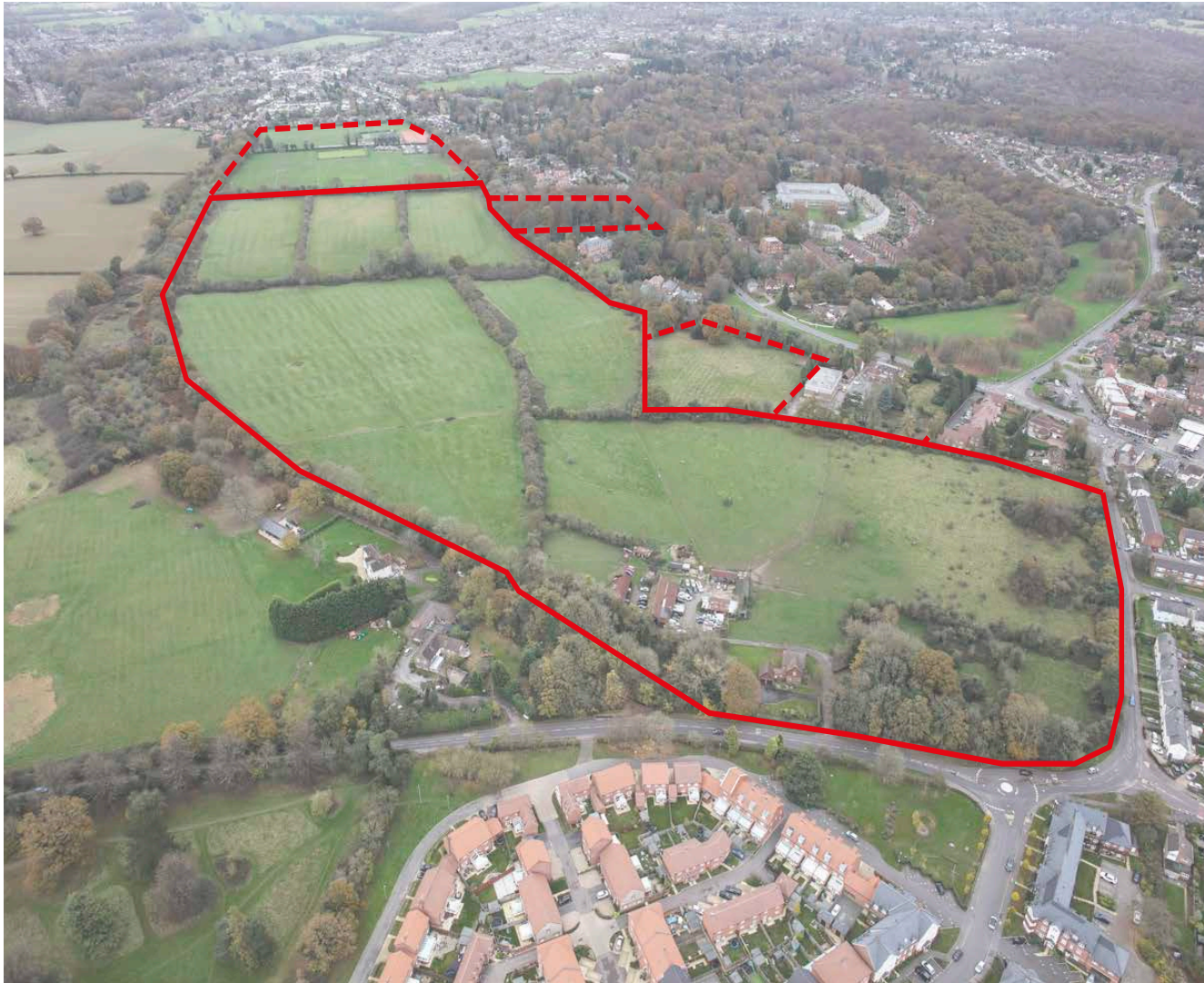
FIG. I.2. - LOOKING EAST ACROSS THE SITE
