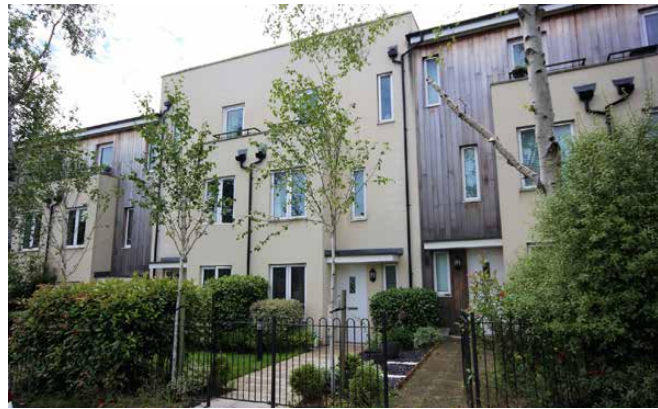
FIGURE 4.22 CONTEMPORARY TOWN HOUSES ON TOTTRIDGE LANE
