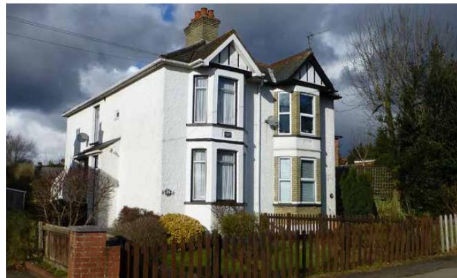
FIGURE 4.24 DETAILING ON RENDER BUILDINGS
